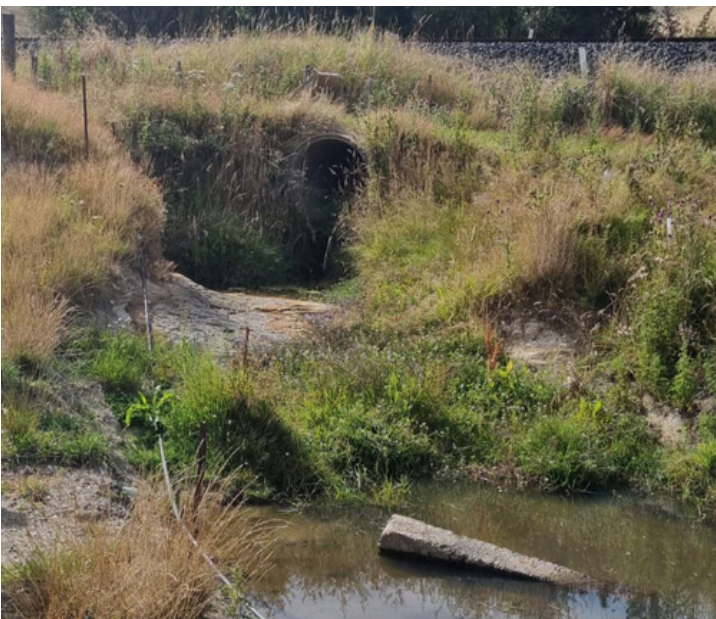
Pre-construction site assessment of perched culvert in the Pleasant River catchment.
